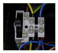
^ 3-way terminal block with built-in fuseholder proved handy
